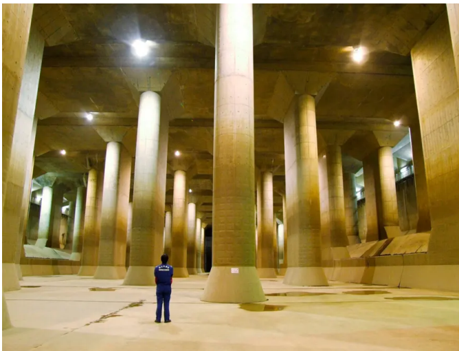
A pressure-controlled water tank in Kusakabe, Japan, constructed to protect Tokyo against floodwaters and overflow of the city's major waterways and rivers during heavy rain and typhoon seasons. Photograph: Ho New/Reuters
